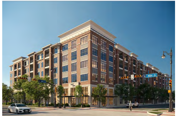
Main and Mill Lofts
