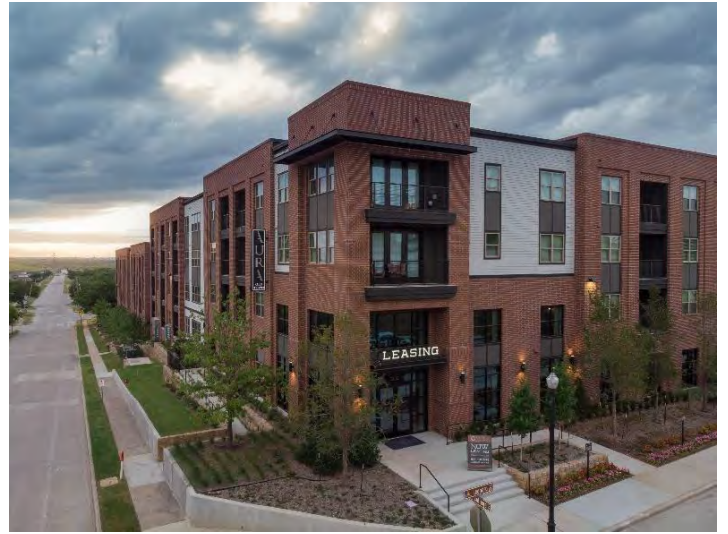
Old Town Station
